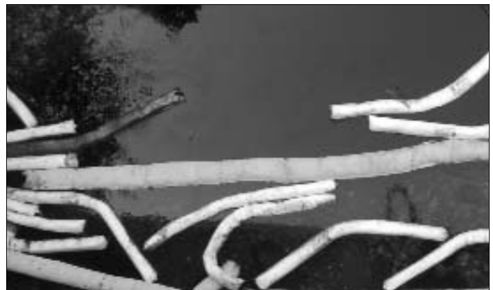
Foam booms and oil-absorbent tubing helped contain the oil spill.
