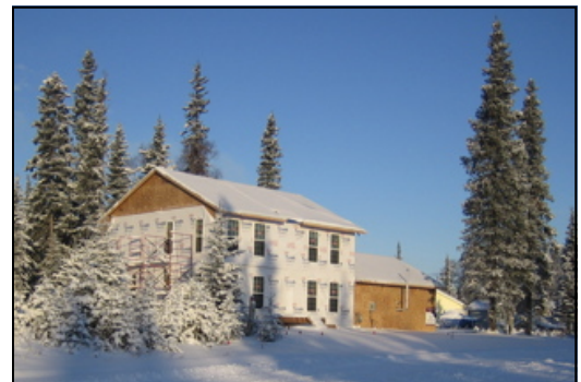
House of Hope '07 Under Construction
