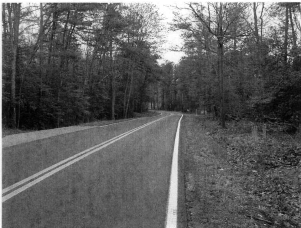
Mile Point 0.7, looking southwest Photo 6 of 7
