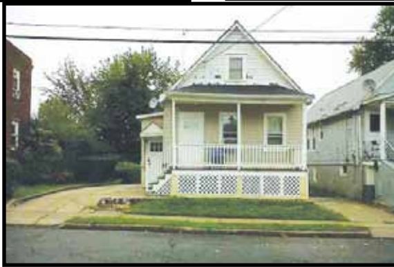
PERTH AMBOY - Nice cozy home, looking for a loving family for some TLC. Huge double lot (50 x 100), 2 detached garages. New piping throughout the home. Don't wait! Will go quickly!!! $99,900
