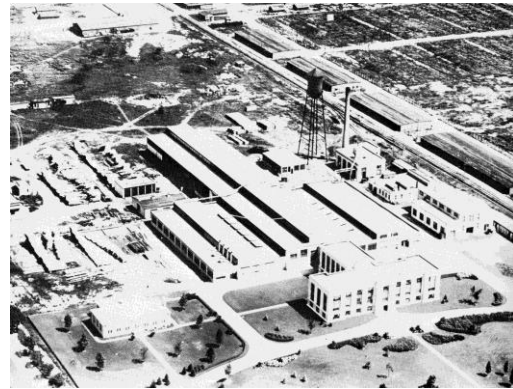
Curtiss Garden City factory, aerial view
