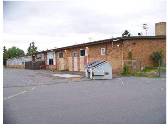
Main building (292A), west (rear) elevation, looking northeast.
