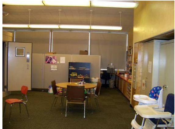
Main building (292A), testing room (originally a classroom), looking west.
