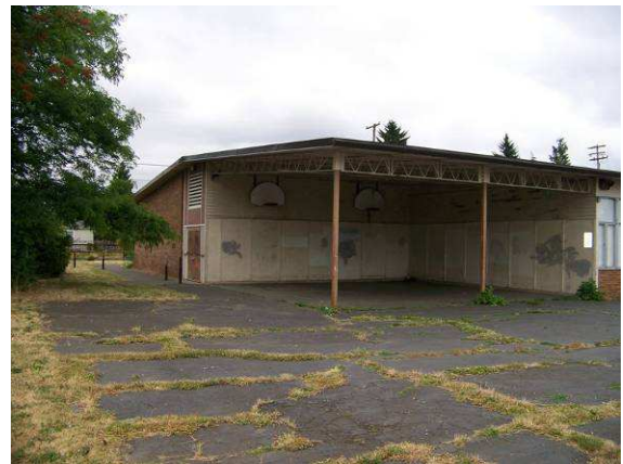
Main building (292A), play court at north (side) and west (rear) elevations, looking southeast.
