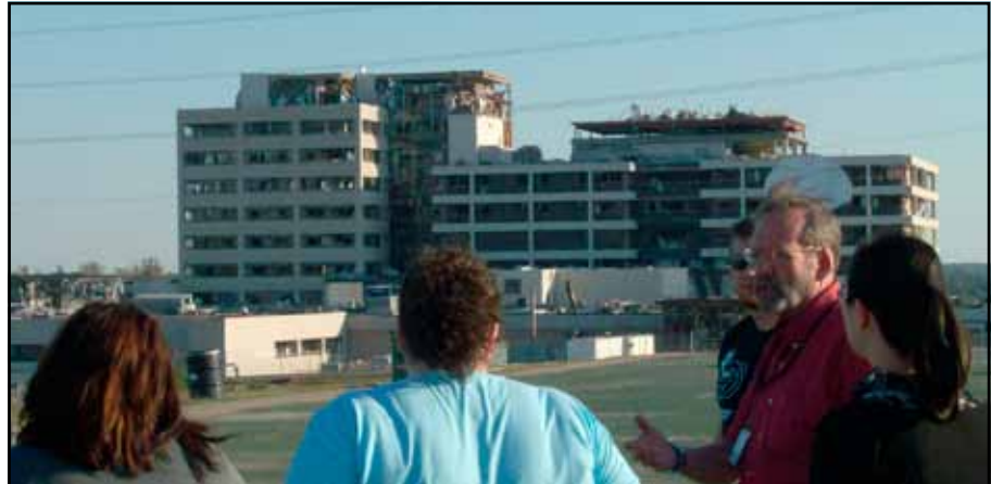
Above, Mr. Stammer pointing out damage to the St John's hospital. Later, students viewed the portable hospital erected to accommodate St. John's patients until the new hospital is built.
