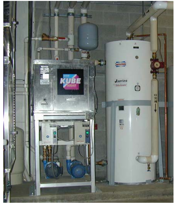
Figure 5. A 10-ton water-to-water heat pump draws heat from the earth loop to produce service hot water (showers and ice flooding) at 120°F (50°C)
