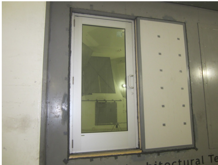
Source Room View of Installed Specimen
