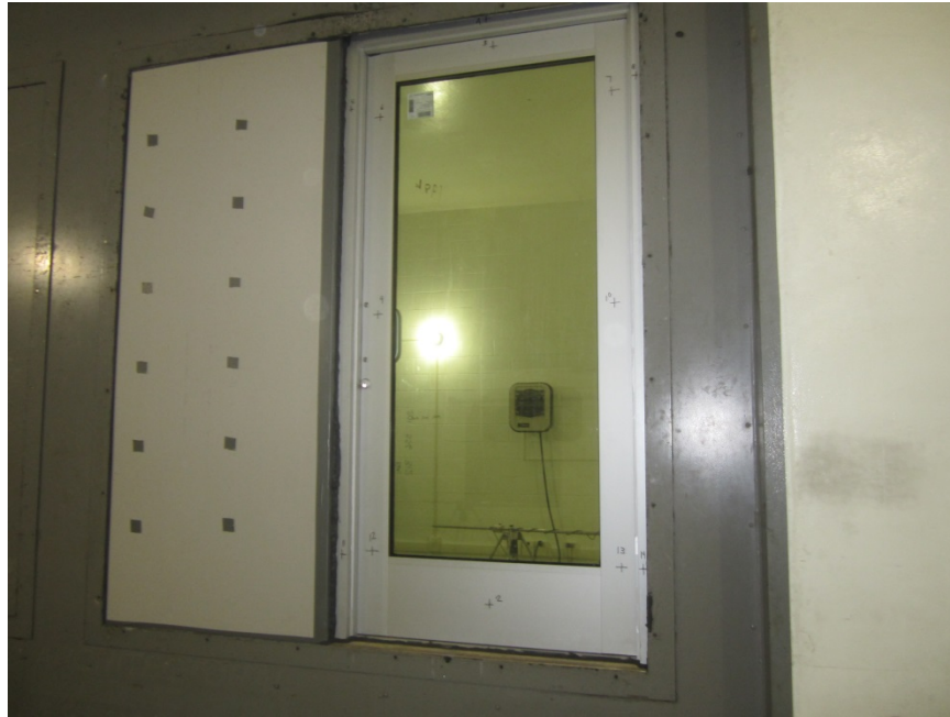
Receive Room View of Installed Specimen
