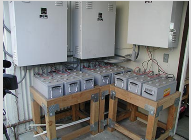
Pictured are cabinets that house three cathodic protection (CP) control units and the respective banks of batteries below them. This control unit operates the photovoltaic-powered CP system. Photo by David Bailey, ERDC-CERL.
