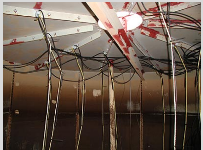
Black cabling for ceramic anodes is hung from the ceiling of the tanks. Yellow nylon ropes secured to the cables have ceramic insulators tied to them at the bottom (providing ballast to the cable). This configuration keeps the anodes suspended vertically in the water to keep them from swaying out of position. Photo by David Bailey, U.S. Army Corps of Engineers, ERDC-CERL.
