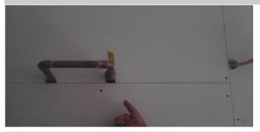
Instead of cutting out an opening in the middle of a sheet for the water heater loop, try doing what is shown in the picture to the left. Cut all of the way across the sheet, even with the bottom of the pipe, and then make two small u-shaped openings in the bottom of the top piece to slip over the pipe. This usually results in a much neater and easier to tape finish job.
