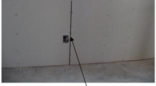
• Avoid joint breaks next to outlets, switches, or edges of windows and doors.
