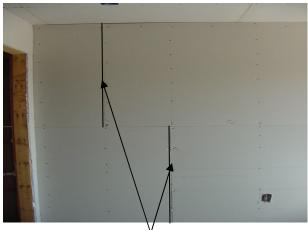
Stagger all butt<sup>y</sup> joints by at least 24".
