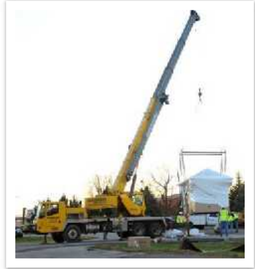
Only necessary employees may be within the fall zone.
