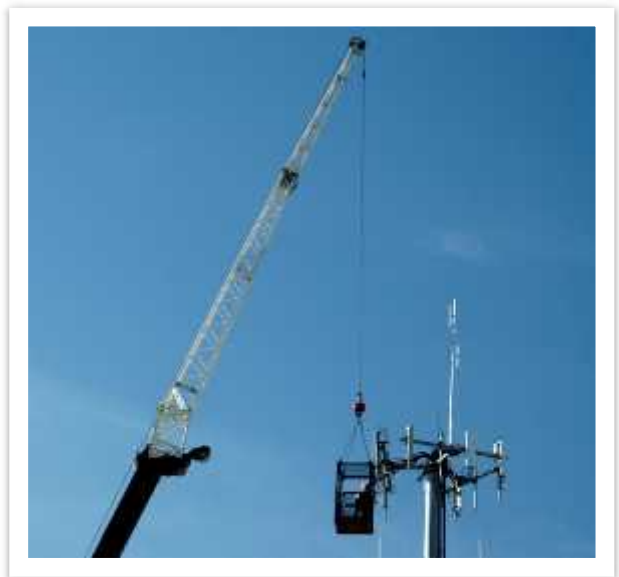
When the occupied personnel platform is in a stationary working position, the load and boom brakes and locking features must be engaged.
