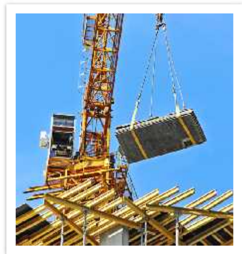
Synthetic slings must be protected from abrasive, sharp or acute edges, and configurations that could cause a reduction of the sling's rated capacity.
