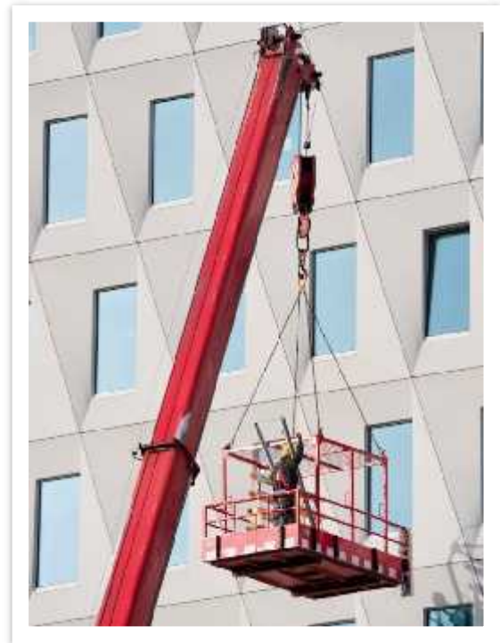
Employees must wear personal fall arrest systems whenever they're occupying a personnel platform.
