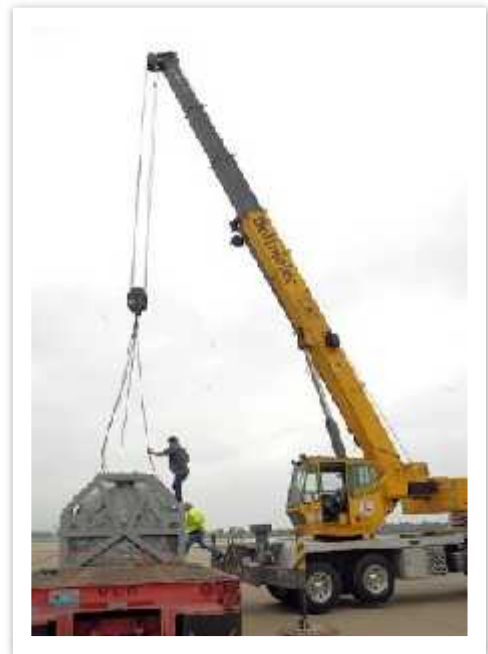
Under most circumstances a personnel platform must be used when hoisting employees.
