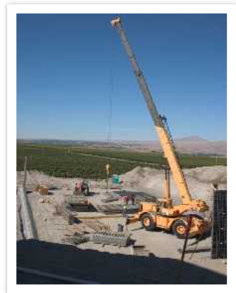
The operator's trainer and the operator-in-training must be in direct line of sight of each other.
