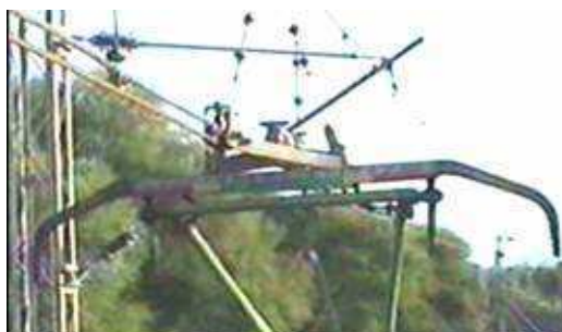
Fig-24 Stagger of section insulator
