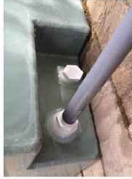
Internal Float Valve System 1" Drain and 1" Line-In Fitting
