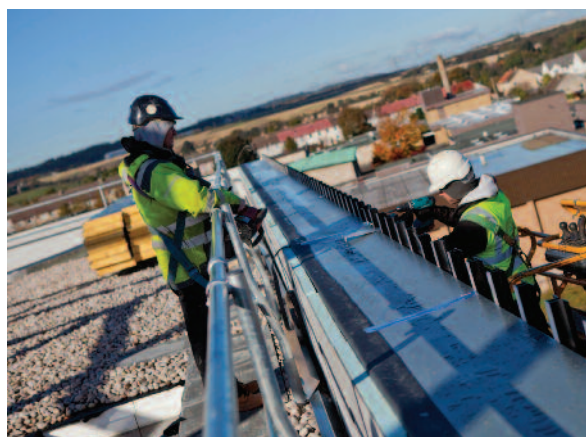
Above: Construction at Wester Hailes Healthy Living Centre.
