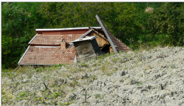
Natural hazards, such as landslides, often cause damage to human property and loss of lives. The picture shows a house damaged by a mud flow in the Buzau County, Romania. (Image distributed by EGU under a Creative Commons licence via www.imaggeo.net . Credit: Raluca-Mihaela Maftei)
