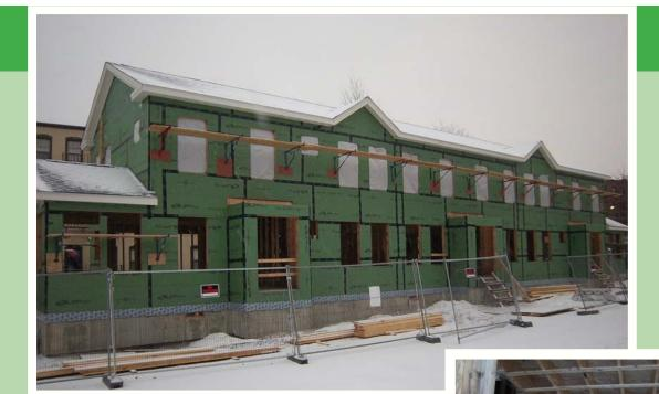
**THE ROOF IS ON!** With the help of volunteers and our Habitat Construction Crew, the Blue Hill Place project was secured and covered just in time for the first snow. The building is fully framed, roofed, shingled, and interior wall partitions have been erected.
