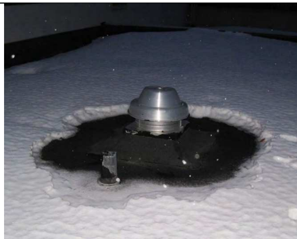
10. Roof Mounted Exhaust Fan, typical
