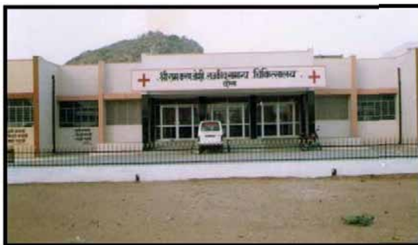
Fig 4: District Hospital Dausa
