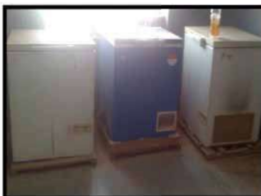
Fig8: Cold chain facility at the DH
