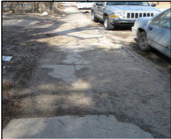
Loss of Curb (Code: C5)
