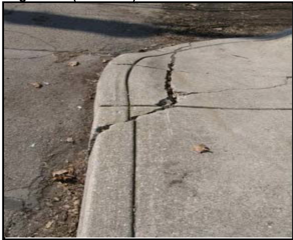
Loss of Curb (Code: C5)
