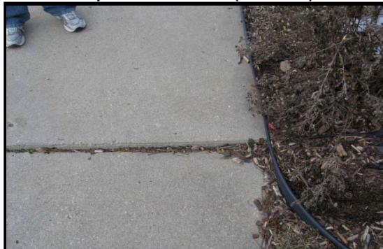
Vertical Displacement > 2Cm (Code: S7)
