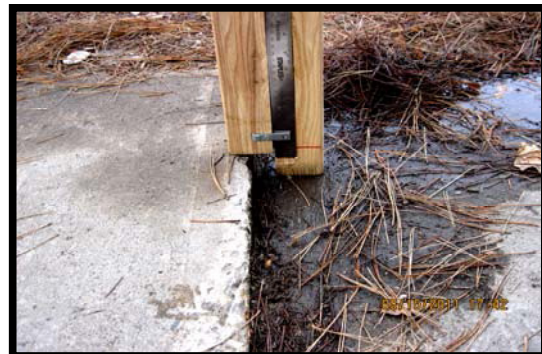
Vertical Displ. > 2Cm (Code: S7) Whitburn St
