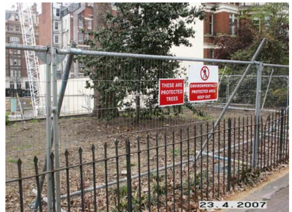
Fencing with signs
