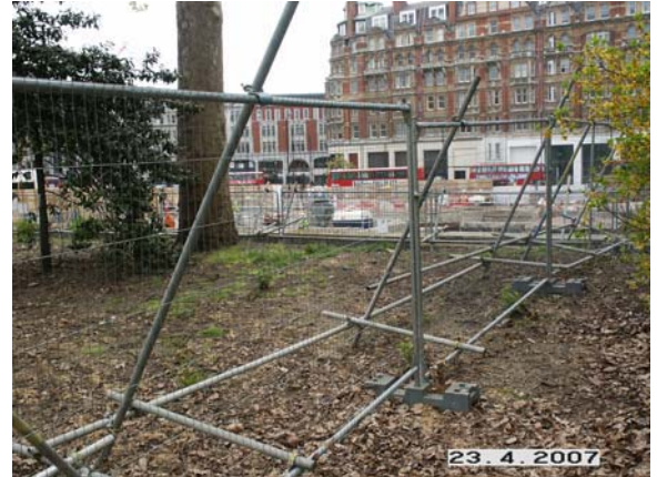
Effective fencing in position
