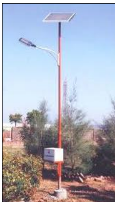
Figure 2.2: Stand-alone PV with battery bank for street lighting
