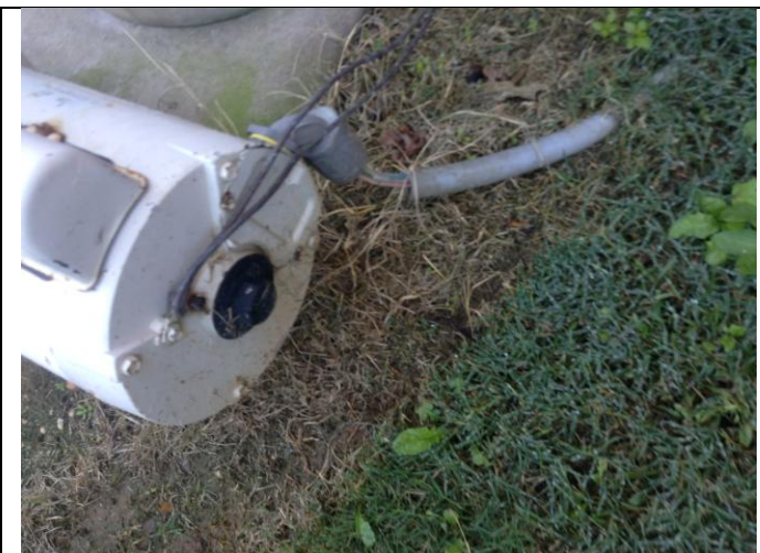
Sample of disconnected conduit at the pool
