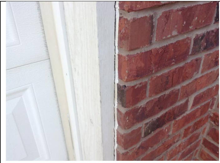
Sample of separation around the garage door frames
