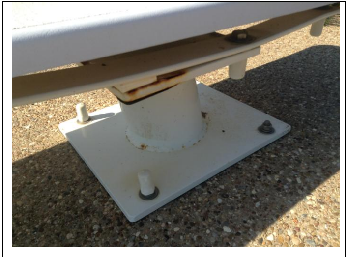
Sample of rust and exposed bolts at the diving board
