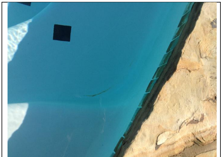
Sample of crack with rust stain in the pool
