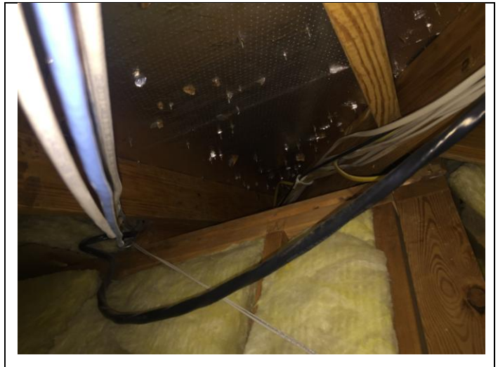
Sample of missing insulation in the attic
