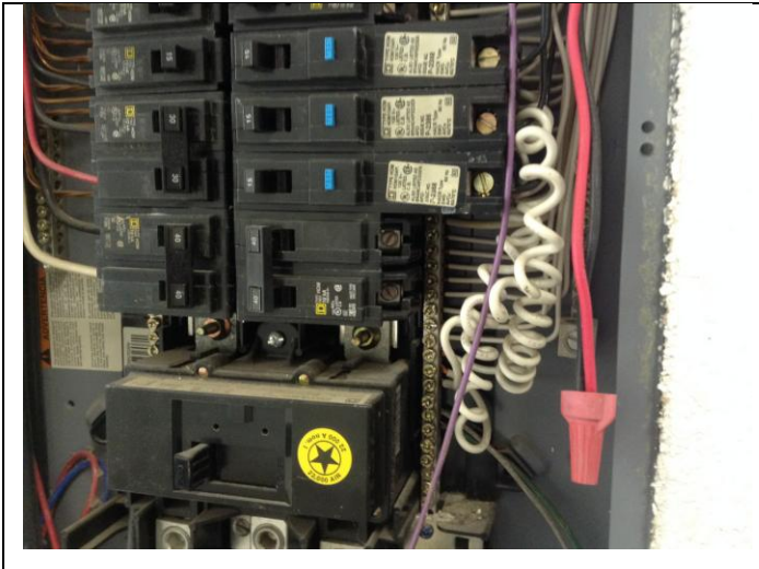
Sample of wire too close to breakers
