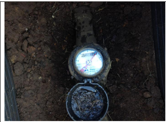
General photo of water meter (no movement at this time)
