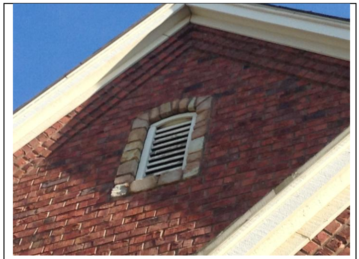
Sample of peeling paint at gable vent
