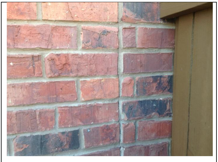
Sample of uneven separation at expansion joint
