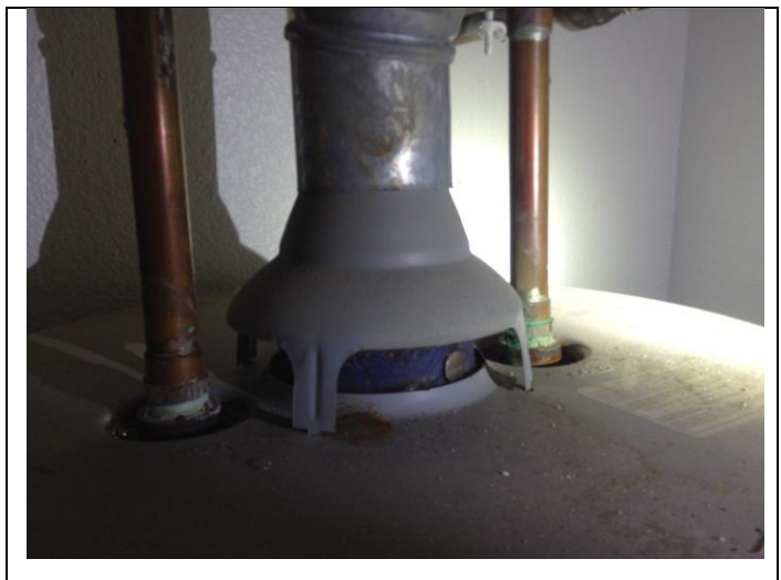
Sample of corrosion on water heater supply fitting
