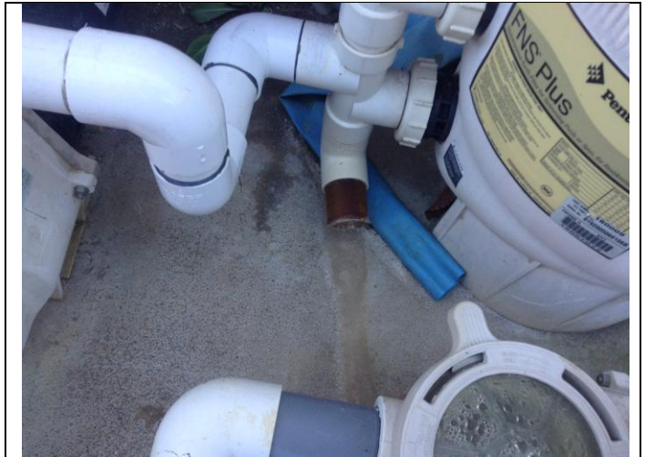
Sample of damaged backwash drain line
