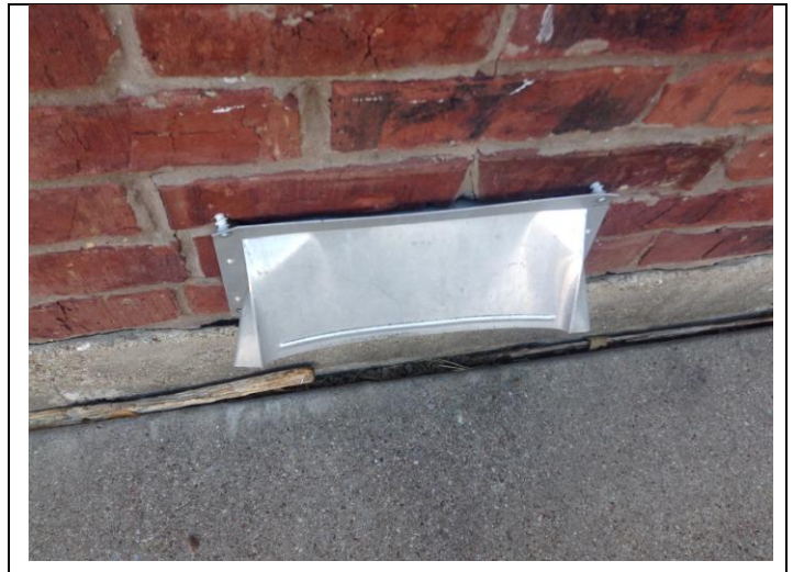
Sample of improper set vent-a-hood exhaust vent cover
