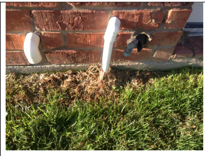
Sample of exposed sprinkler control wires at damaged conduit
