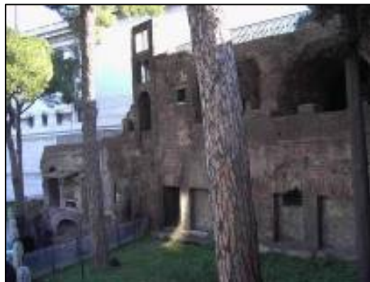
Remains of a multi-level insula (island) near the Capitoline (Rome), which housed non-elite families.
