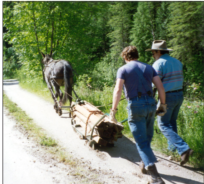
Figure 33—Fremont grader being used to haul waterbar materials. The grader blade has been removed.
