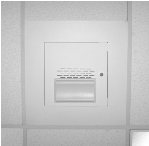
24x24x8 MIMO Ceiling Tile Enclosure – Installed in Ceiling Tile Grid Displayed with a TerraWave 802.11n Dual Band 2.4/5 GHz 2.5/4.5 dBi Ceiling Mount MIMO Omni Antenna and a Cisco 1252 Access Point
