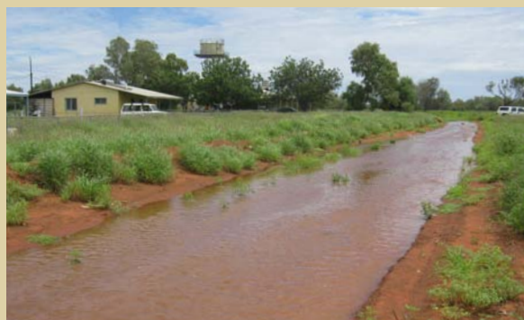
The new drain diverting floodwater at Wilora in 2015.
