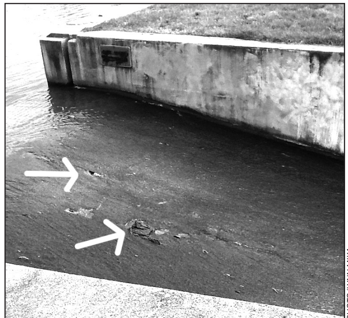
The Main Dam spillway erosion.
