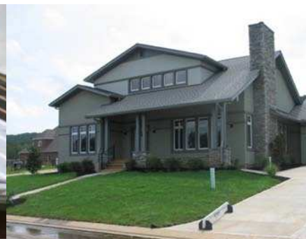
New roof decking, membrane, and shingles are installed over the IRV for a roof that is insulated and ventilated to minimize attic heat build up.
