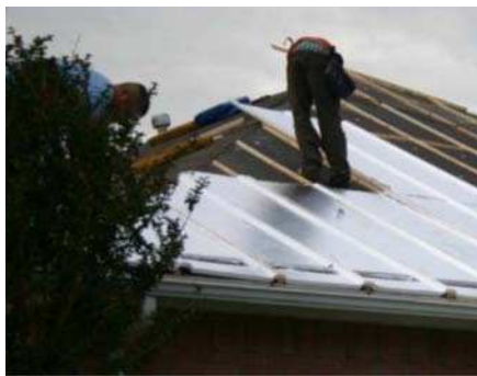
Roofers installed the insulated and ventilated roof deck over an existing roof in this retrofit application in Oak Ridge, Tennessee. The EPS is installed on furring strips attached to the existing shingles.
