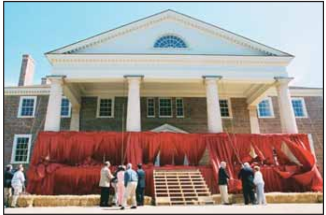
John F. Macon helps to pull ropes revealing the restored portico. Photo by Richard Robertson, courtesy of the Montpelier Foundation.
