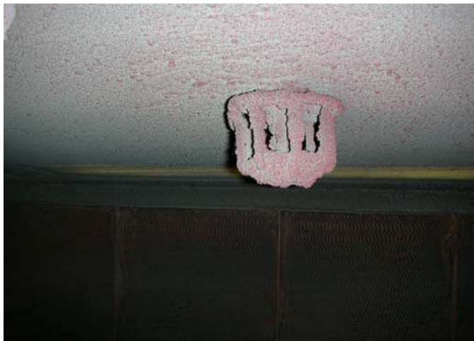
Loaded Sprinkler in Head Cage Head
