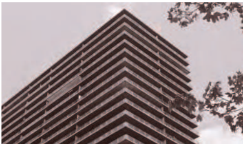
Jeffersonian Apartments Detroit, MI [ BELOW ]
