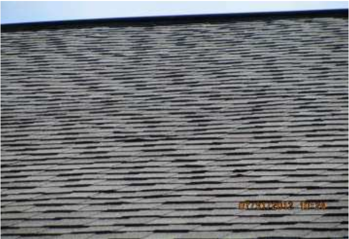
Roof Field Asphalt-Fiberglass Shingles - No Sagging
