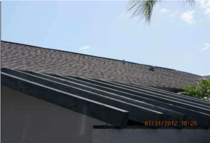
Front Elevation Asphalt-Fiberglass Shingles - No Sagging
