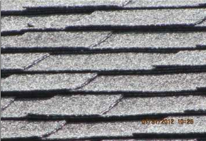
Asphalt-Fiberglass Shingled Roof No Curling or Deterioration
