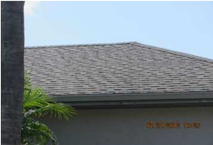
Roof Field Asphalt-Fiberglass Shingles - No Sagging
