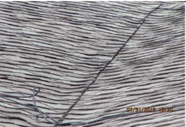
Roof Valley Asphalt-Fiberglass Shingles - Closed Flashing
