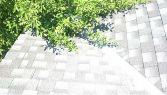
Trim back trees and shrubs away from home.
