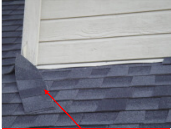
Shingles blowing off on the west side of the home.
