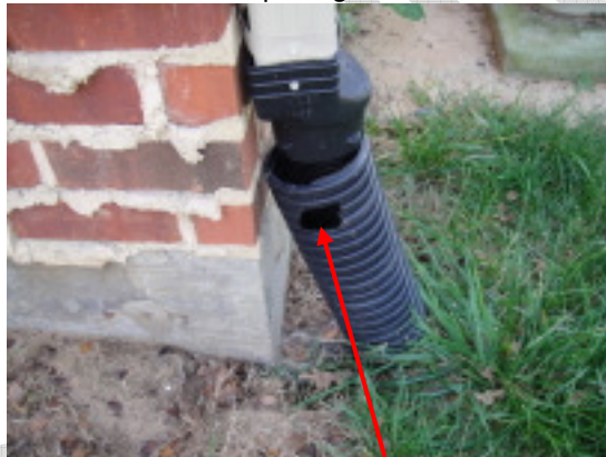
Some of the gutter downspouts have pulled loose from the underground drain pipes
