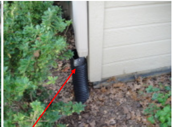
Some of the gutter downspouts have pulled loose from the underground drain pipes
