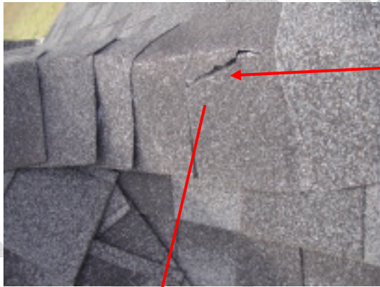
Shingles blowing off on the west side of the home.
