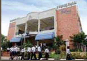
Hebron Hall - Indoor Stadium
