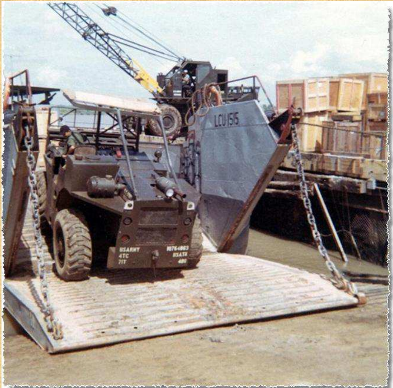
Rough Terrain Cargo handler (forklift) loading LCU
