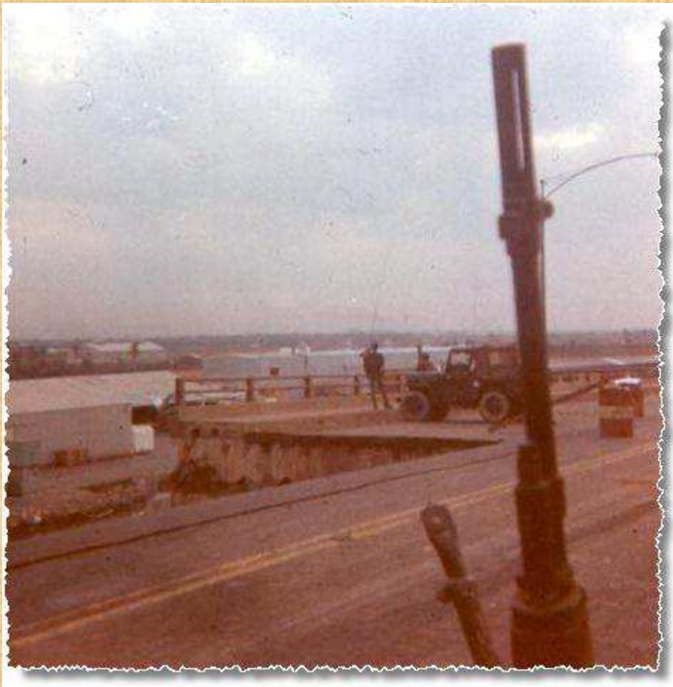
missing section of bridge at QLI over Saigon River at Newport
