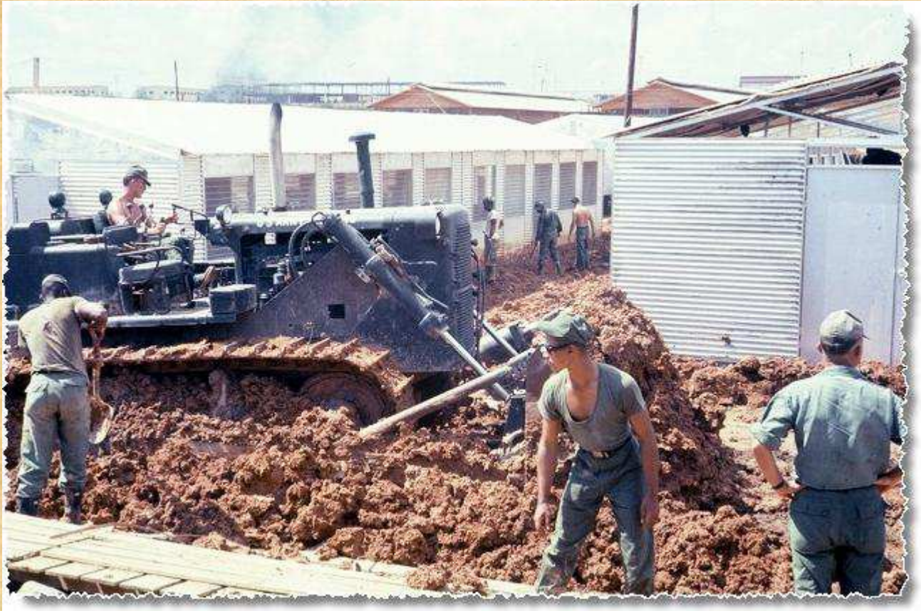
Construction for metal huts (and the mud)
