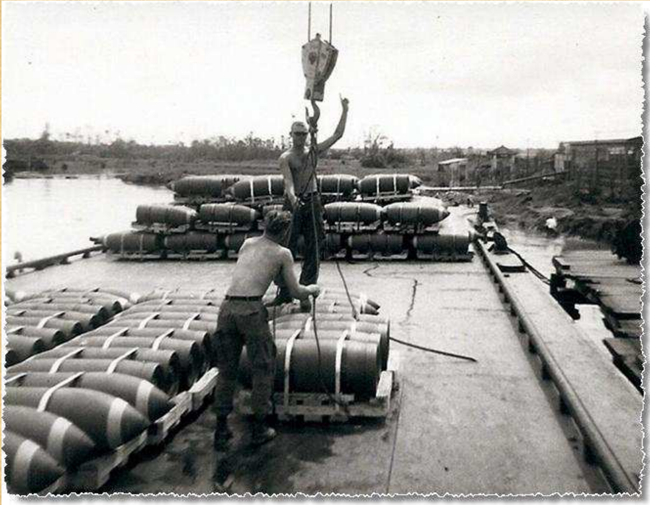
Rigging projos for crane movement
