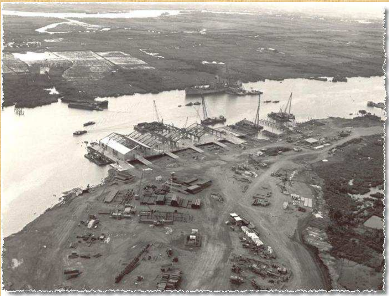
Newport warehouses under construction
