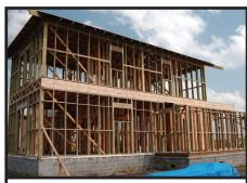
Advanced framing - larger lumber, but wider spacing and stack framing provides strength and more insulation with fewer studs and lower framing cost.
