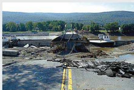
River bridge destroyed by heavy flooding.
