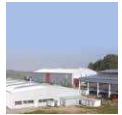
FieldTurf Fiber Production Plant - Absteinach, Germany
