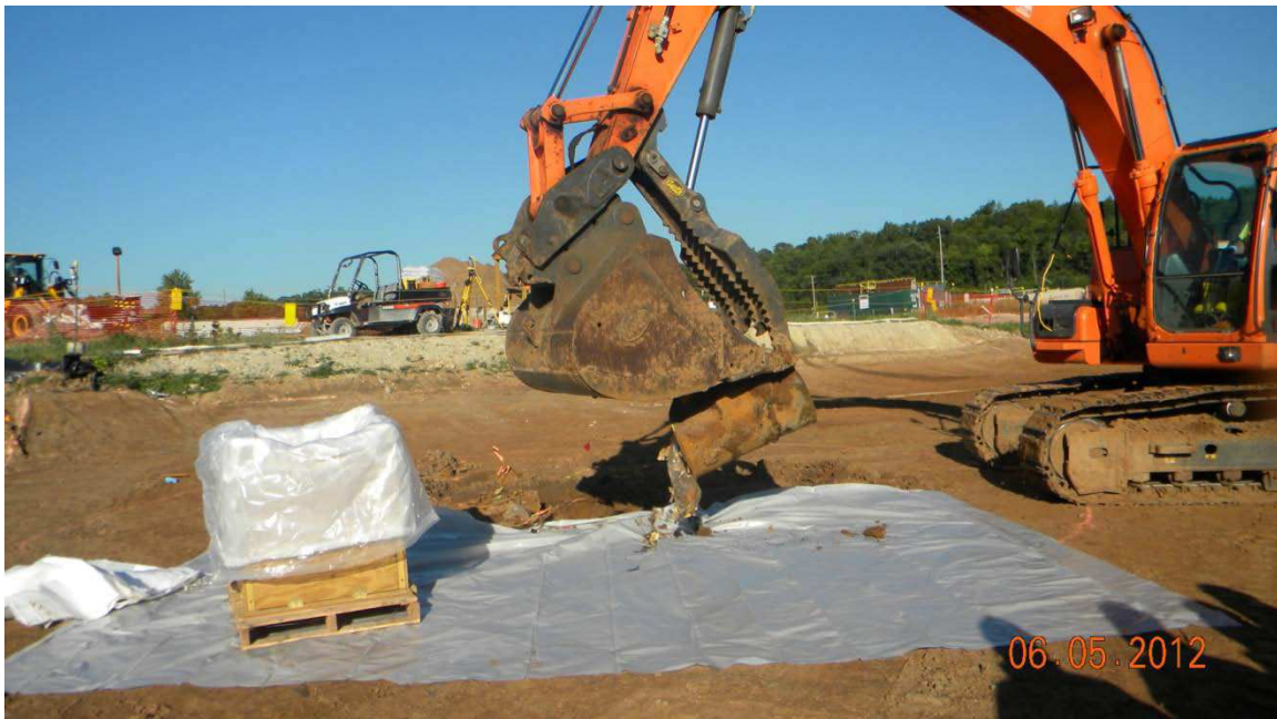
Photo #2 Opening and Dumping Drum
