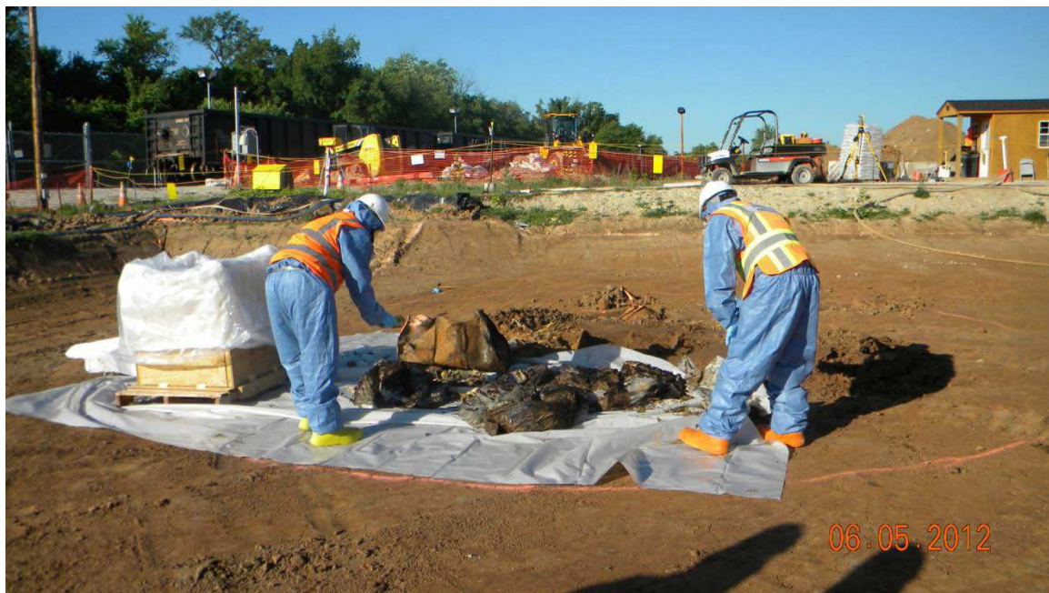
Photo #3 Surveying and Sorting Drum Contents
