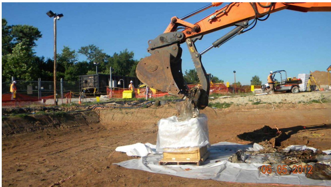
Photo #4 Loading Waste into Waste Transport Container
