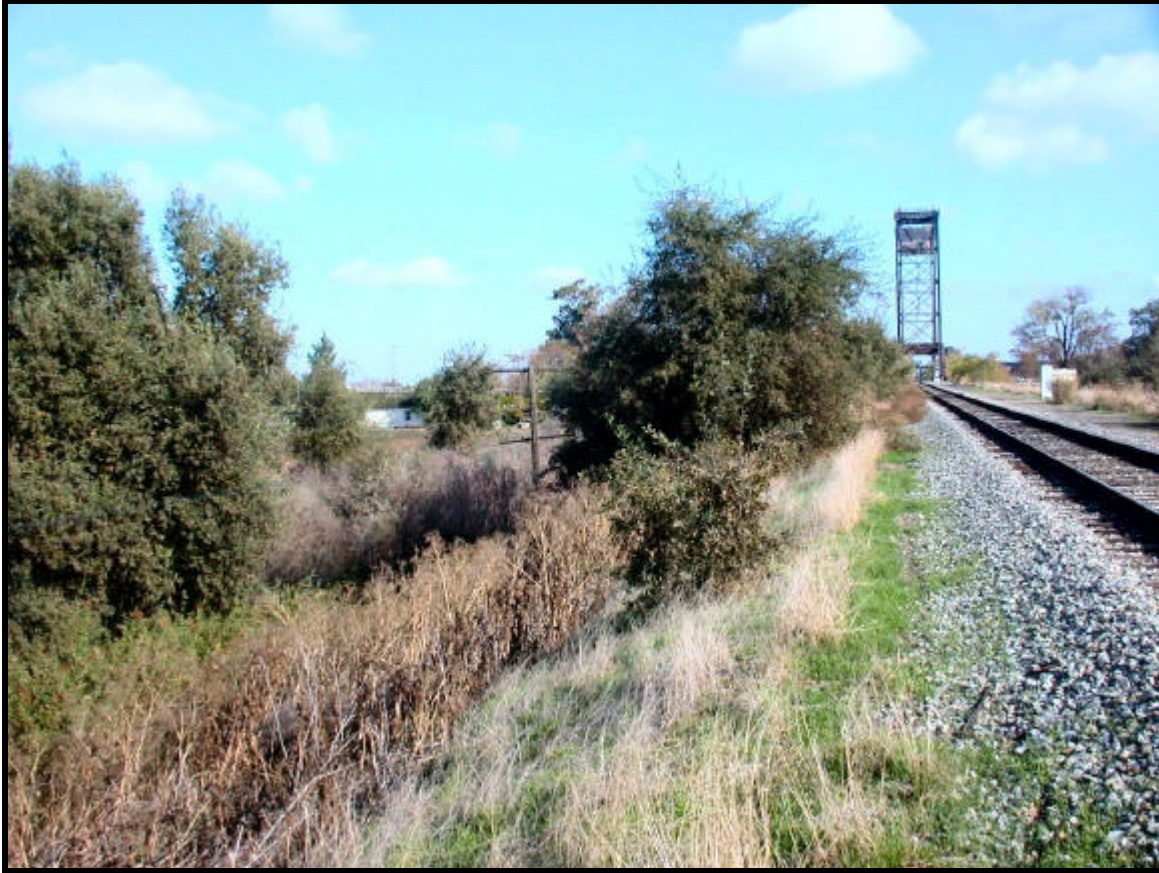
Figure 4. Photograph of the Southern Pacific Railroad bed and north-side right-of-way, facing eastward, on Stewart Tract. The larger, darker-colored trees are Valley oaks; willows, wild roses, blackberries, and other woody and weedy plants grow in the borrow pits along the bases of the railroad embankments. Riparian brush rabbits are found intermittently along the railroad where there is sufficient habitat for home ranges (photo by D.F. Williams).
