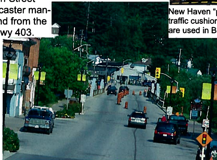
A traffic light lane restriction manages the flow of traffic while permitting two way traffic access.
