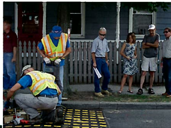
New Haven "puts the brakes on drivers" with traffic cushions that slow traffic to 30k. These are used in Burlington Ontario as well.
