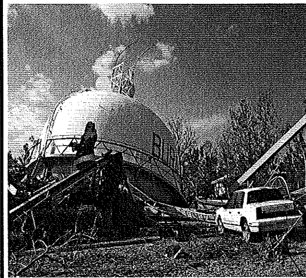
Caption: another view of collapsed water tower
