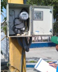
Meter assembly – direct type
