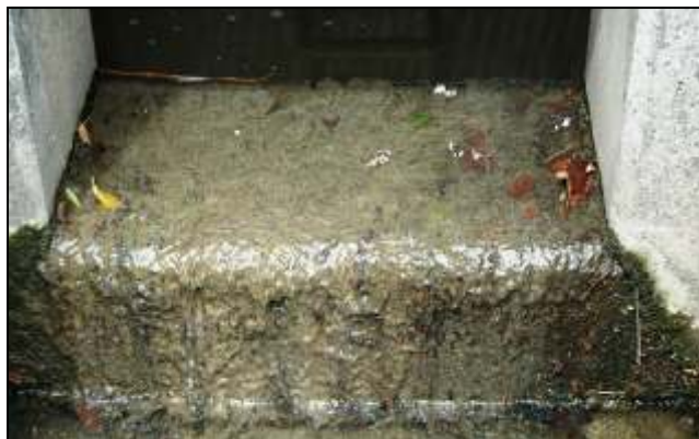
Natural Biofilm Growth on concrete drain
