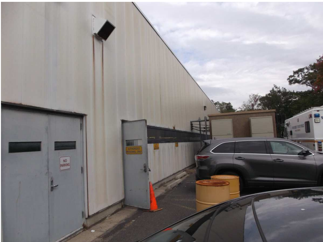
Exterior Panel Discoloration and Rusting at Penetrations
