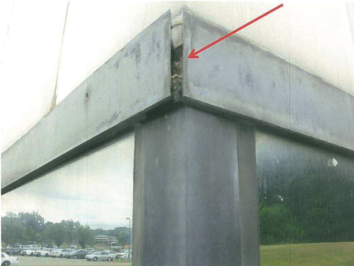
Photo No. 07-Open Corner Flashing Joints at Exterior Strip-Windows
