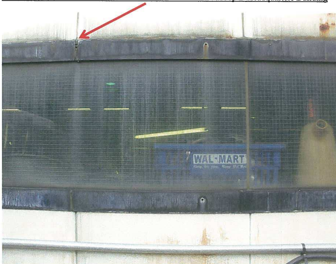
Photo No. 08- Open Joints and Moisture Damage at Tempered Wire Windows
