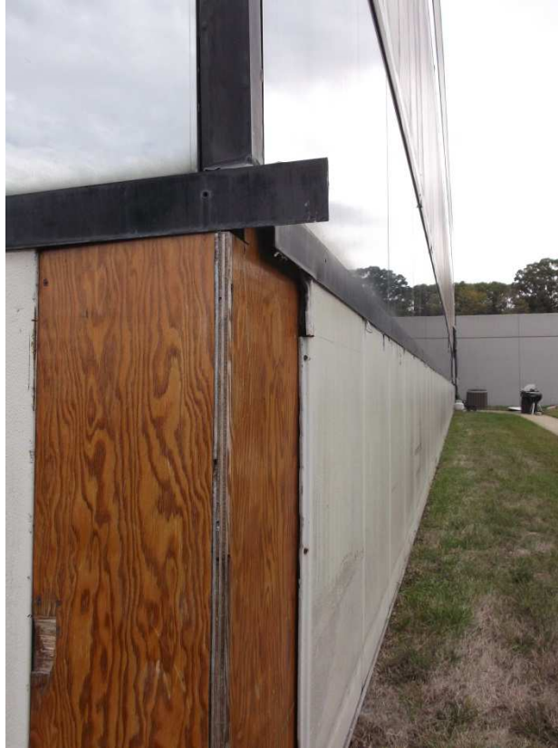
Window Joints and Flashing Failure
