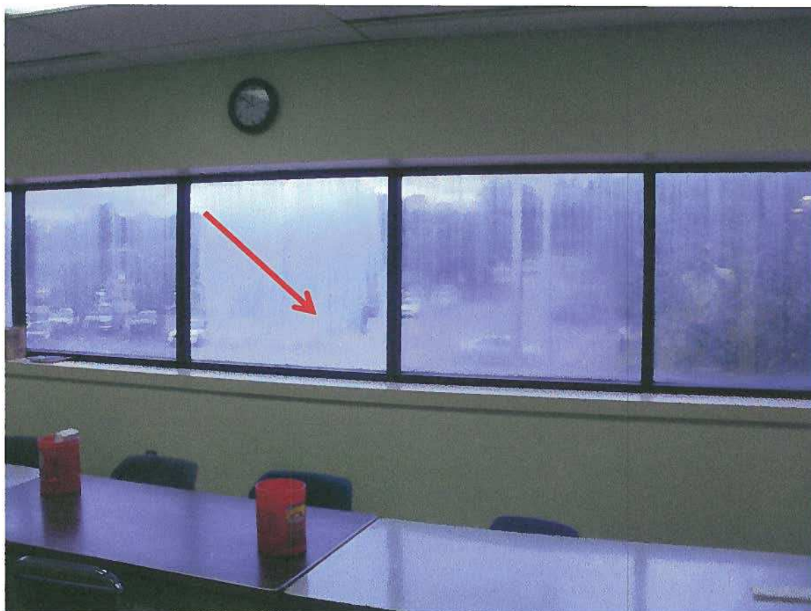
Photo No. 5- Moisture Intrusion between Double Pane Exterior Windows
