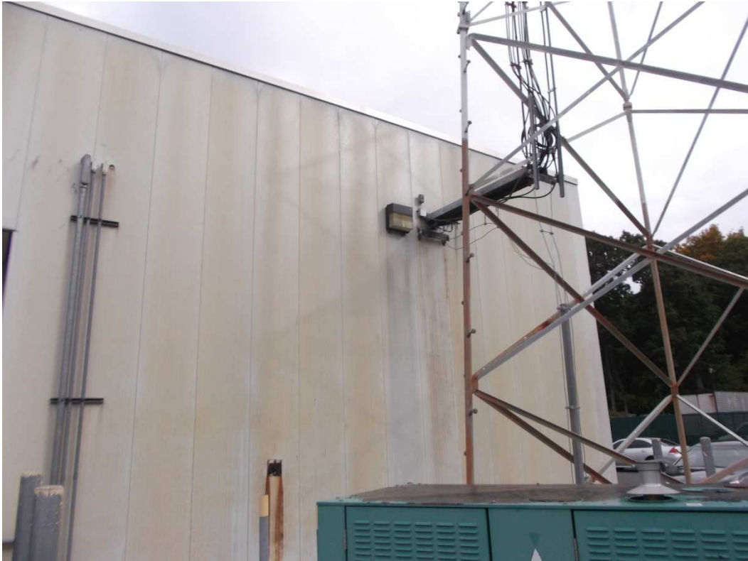
Exterior Panel Discoloration and Rusting at Penetrations
