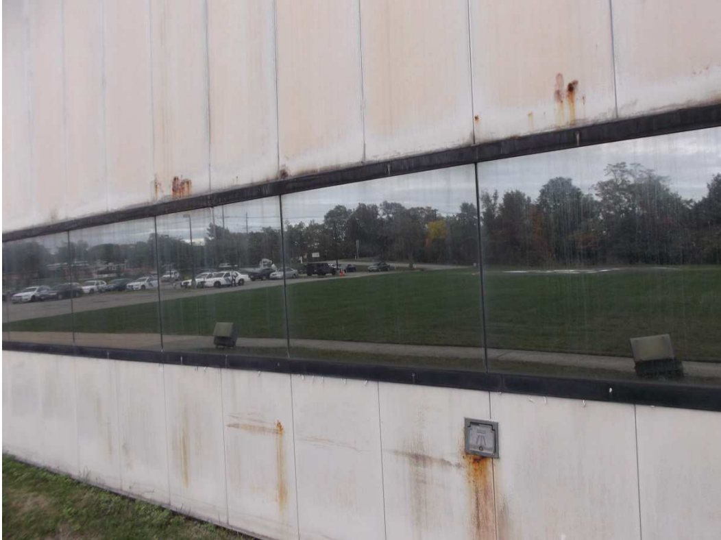
Deterioration/Discoloration of Exterior Wall Panels
