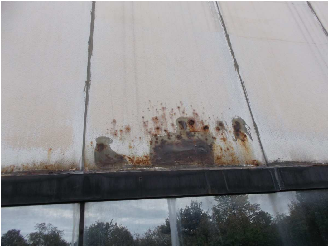
Deterioration/Discoloration of Exterior Wall Panels
