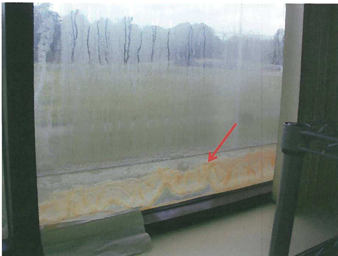
Photo No. 06-Discoloration and Moisture Intrusion between Double Pane Windows
