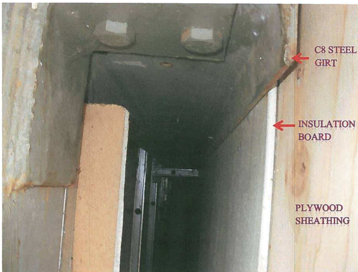
Photo No. 02-Typical Exterior Wall Construction
