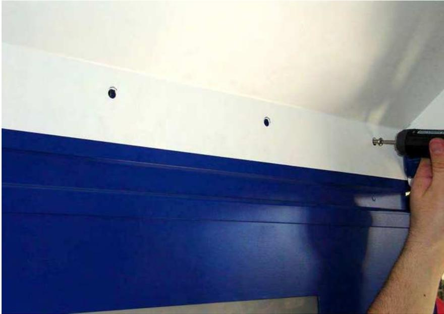
17. Using 7 button-head, 1/2" security screws, screw the Seat Unit Top to the Seat Unit. Some shifting may be required in order to properly align the holes.
