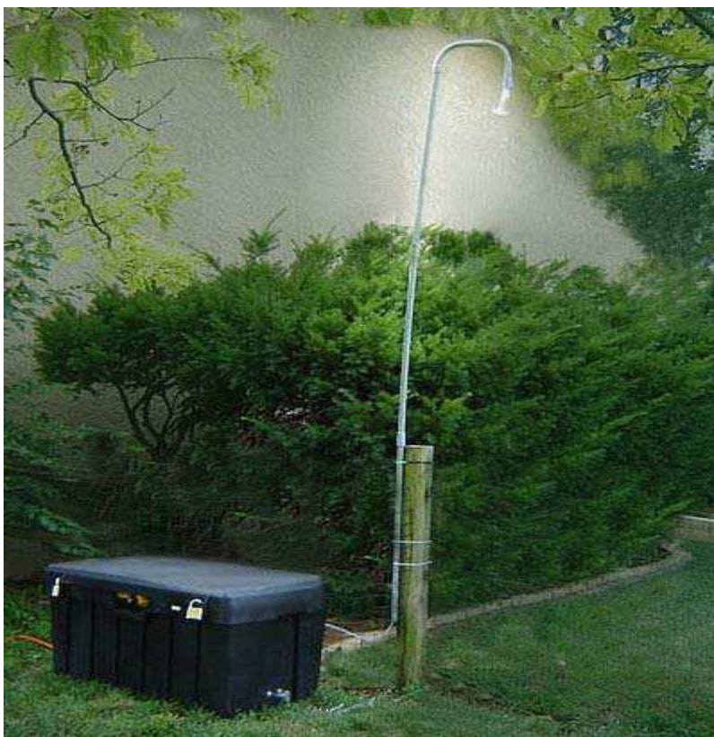
Figure 8. Site 4 Equipment and Setup
