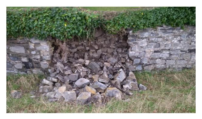
The wall section collapsed across an area approximately 5.0 meters wide X 2.5 meter height X 1.5 meters deep (contractor to determine site dimension of affected areas). The affected limestone Gate Pillars and loose cut stone capping is approximately 30 meters from this area. All organic material must be cut back to ensure reinstatement of capping finish all along the top of the Ha Ha wall. It may be advisable to inspect the entire area
